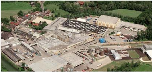
S. Spitz Beverages Factory, Austria ECOTHERM Stainless Steel High Capacity Water Heaters
