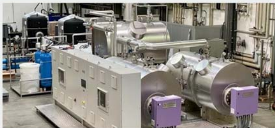
Food & Beverage Factory, Netherlands ECOTHERM Turnkey Electric Clean Steam Boiler, 4.000 kg/h
