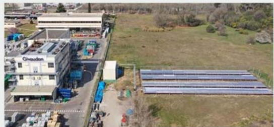
Givaudan Chemical Industry, Spain ECOTHERM Turnkey Solar Steam System
